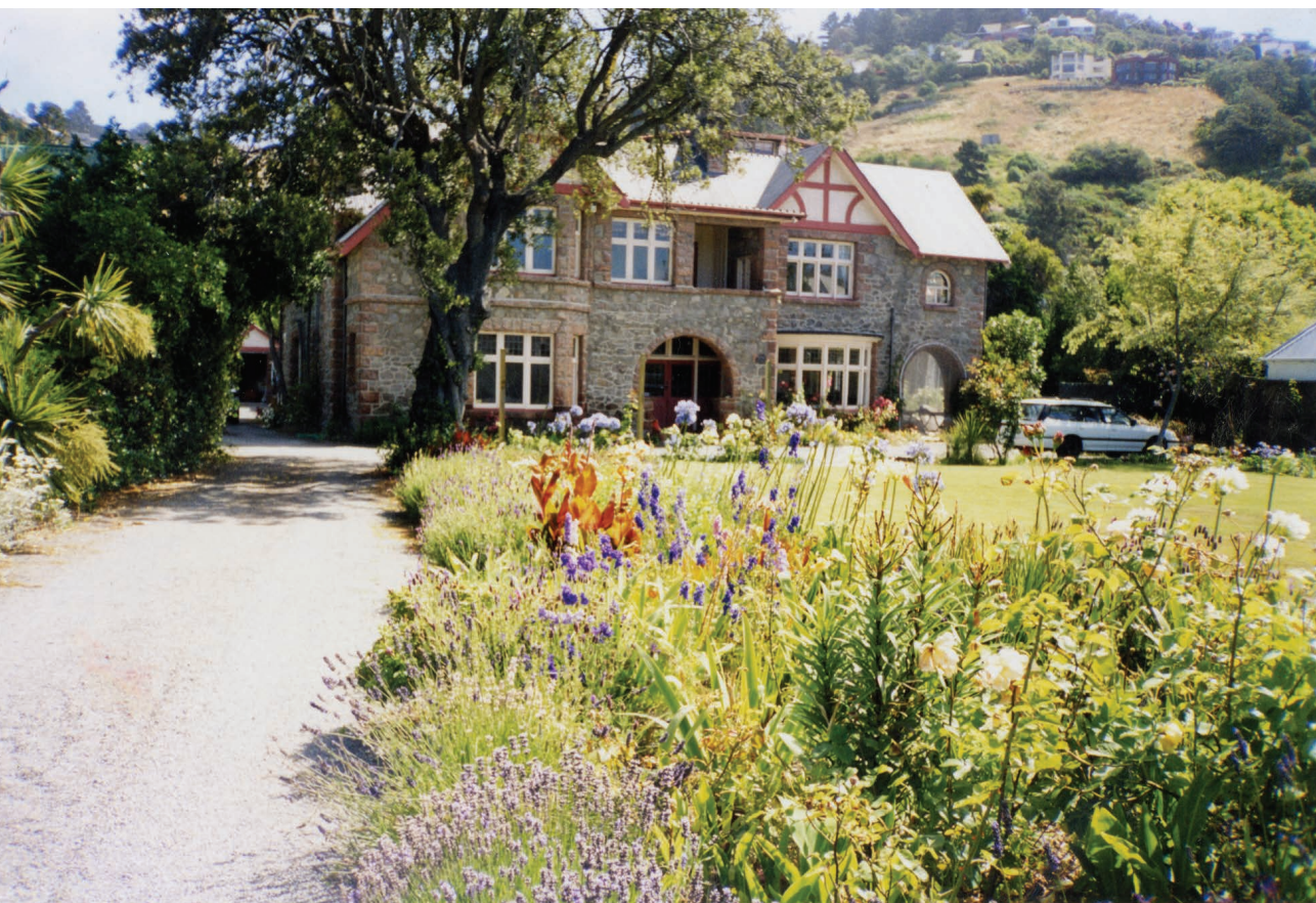
'Rock Villa', Sumner. Photographed pre-earthquakes.
